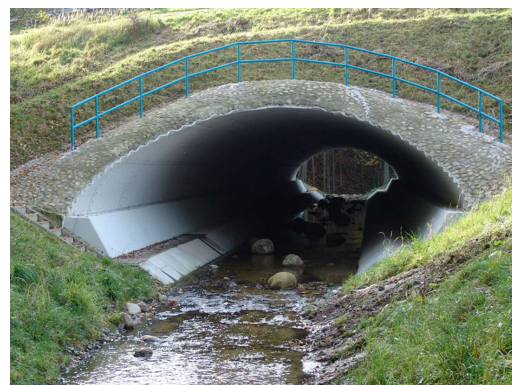
Picture 4: Completed corrugated steel pipes
