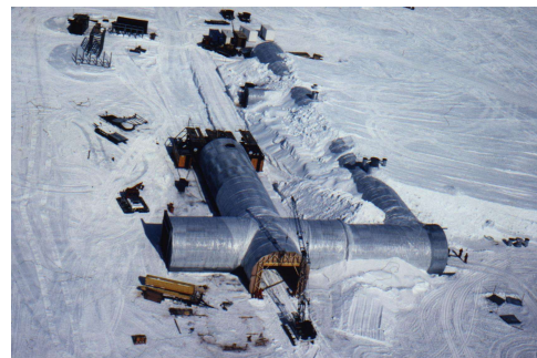
Picture 2: Second Antarctica research station (repeated crossing of circular profiles, span 8,00 m each)
