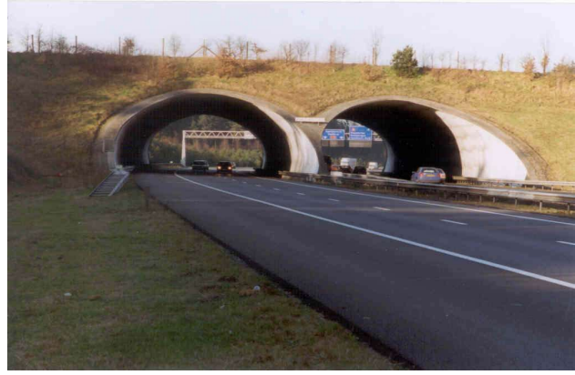
Picture 4: Greenbridge national park Woeste Hoeve (NL) at finale state
