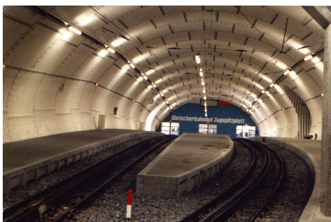
Picture 1: Mountain railway station at the Zugspitze (span 14,22 m)
