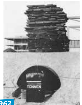
Large-scale load carrying test (> 1000 tons)
