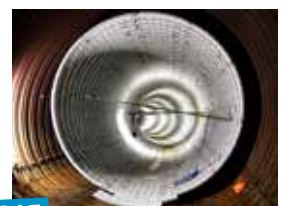
Rebuilding of tunnel with LinerPlate
